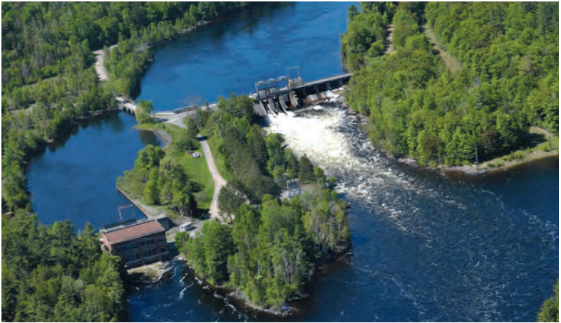
Upper left: The old power plant, built in 1917, is one of OPG's oldest plants and was due for refurbishing. A 2018 tornado spurred the decision to completely redo the plant, rather than refurbish it. Upper Right: The new power plant is the pride of OPG. Built 50 metres upriver with reshaped forebay and tailrace. It generates double the power with the same amount of water.
