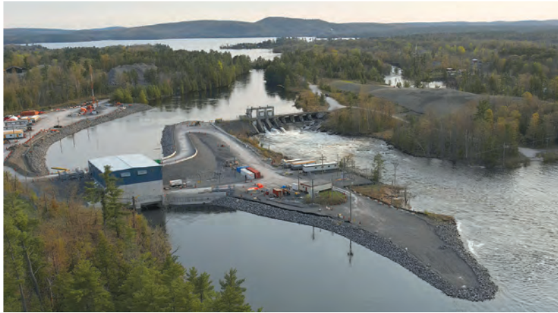
Upper left: The old power plant, built in 1917, is one of OPG's oldest plants and was due for refurbishing. A 2018 tornado spurred the decision to completely redo the plant, rather than refurbish it. Upper Right: The new power plant is the pride of OPG. Built 50 metres upriver with reshaped forebay and tailrace. It generates double the power with the same amount of water.
