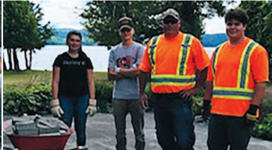
The work crew who built the accessible ramp and the beautiful new patio. L-to-R: Makayla Whyte, Parker Mulvihill, Stephan McDonald, Supervisor, Xander McDonald
