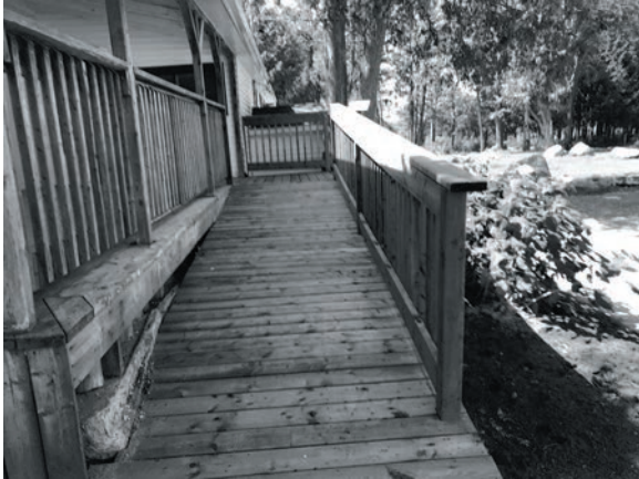
New ramp at Barnet Park Cottage
