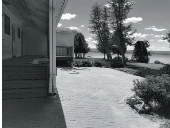
New interlock brick patio at Barnet Park Cottage
