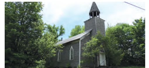
Vennachar Community Memorial Church Closed, but was restored in 1987. A sign says "Visitors inquire at Vennachar Store". The store is now closed.
