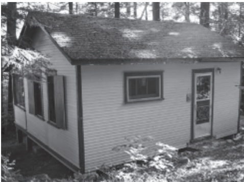
The Alladin, built in 1928 still stands and is used today.
