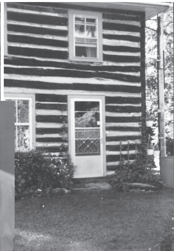
My old log home still stands about 3 miles outside of where Black Donald once was on the Madawaska River. It's a little closer to the water now, after the town was flooded 50 years ago.
