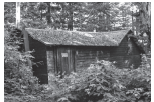
A kitchen with a woodshed on the back was built around 1930. It is used today as a workroom.
