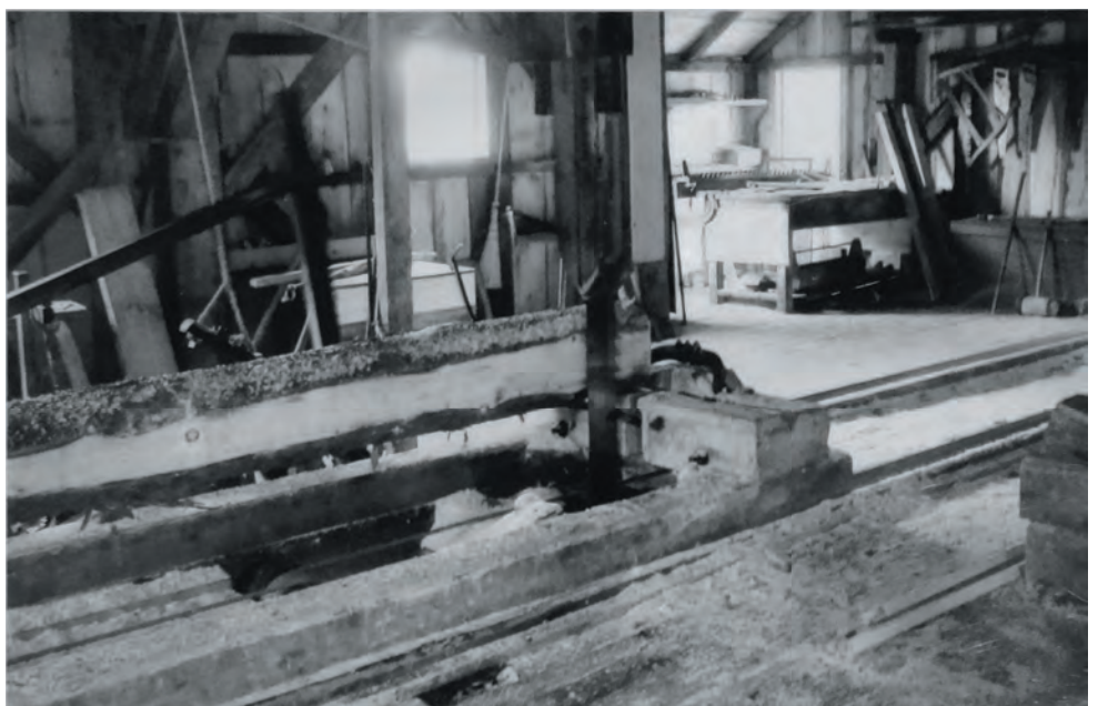
This image is of an old sawmill like that of William Strong's. The long saw blade is set vertically (in the middle of the pic).
