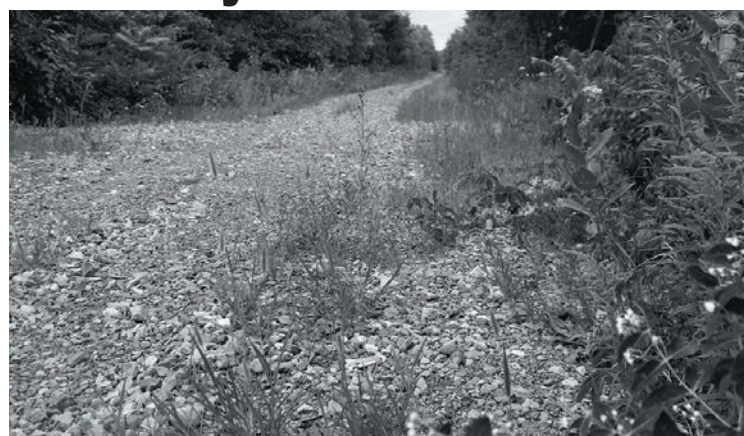
Track ballast is only good as a track bed to support railway ties, and it's a far cry from what is needed on a multi-use trail. It makes a good route, but the surface is almost unpassable
