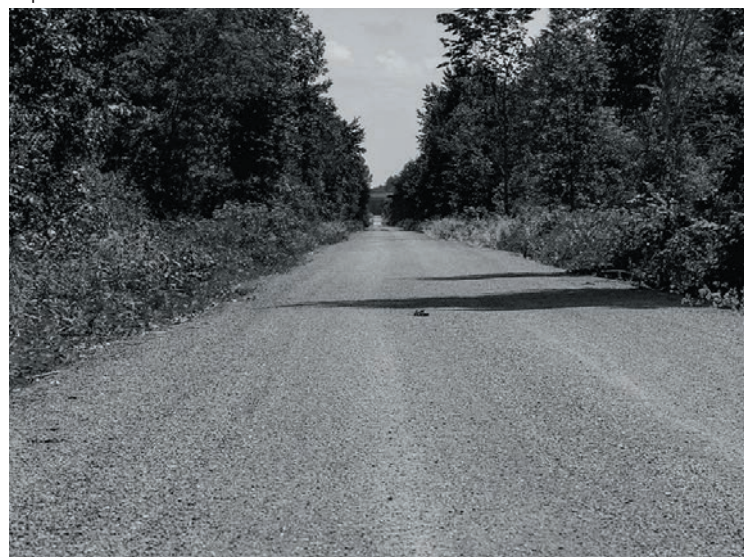
In a few short years, the OVRT has gone from a dream and purchase from CP Rail, to a section of 94 continuous kilometers of firm, smooth stone dust surface.
