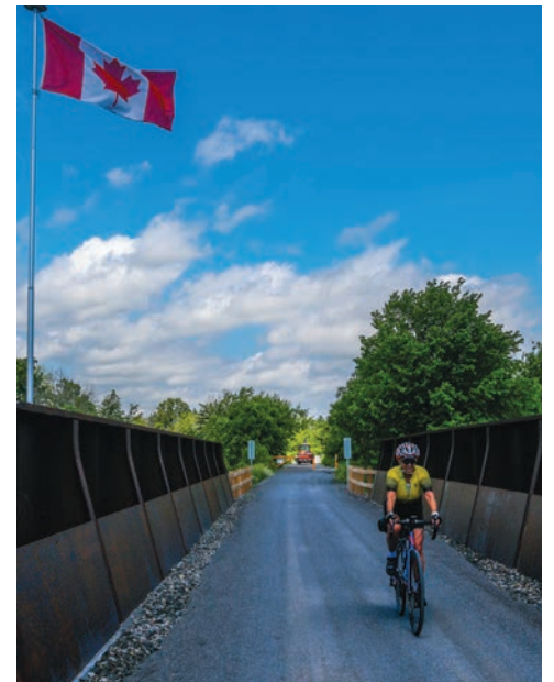
Above: Bridge at Pakenham
