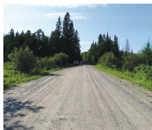
White Bridge today is just a culvert. Trees and brush hide the water on either side.
