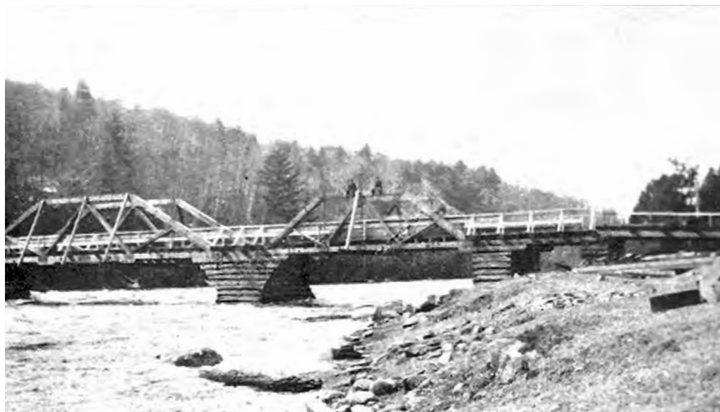
Old photo of the bridge over the Madawaska, formed with original pine and river stone as the base
