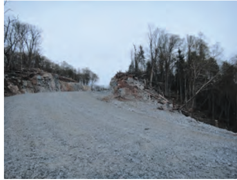
Huge turbine parts can't do ups, downs, twists and turns, so they get levelled and smoothed.
