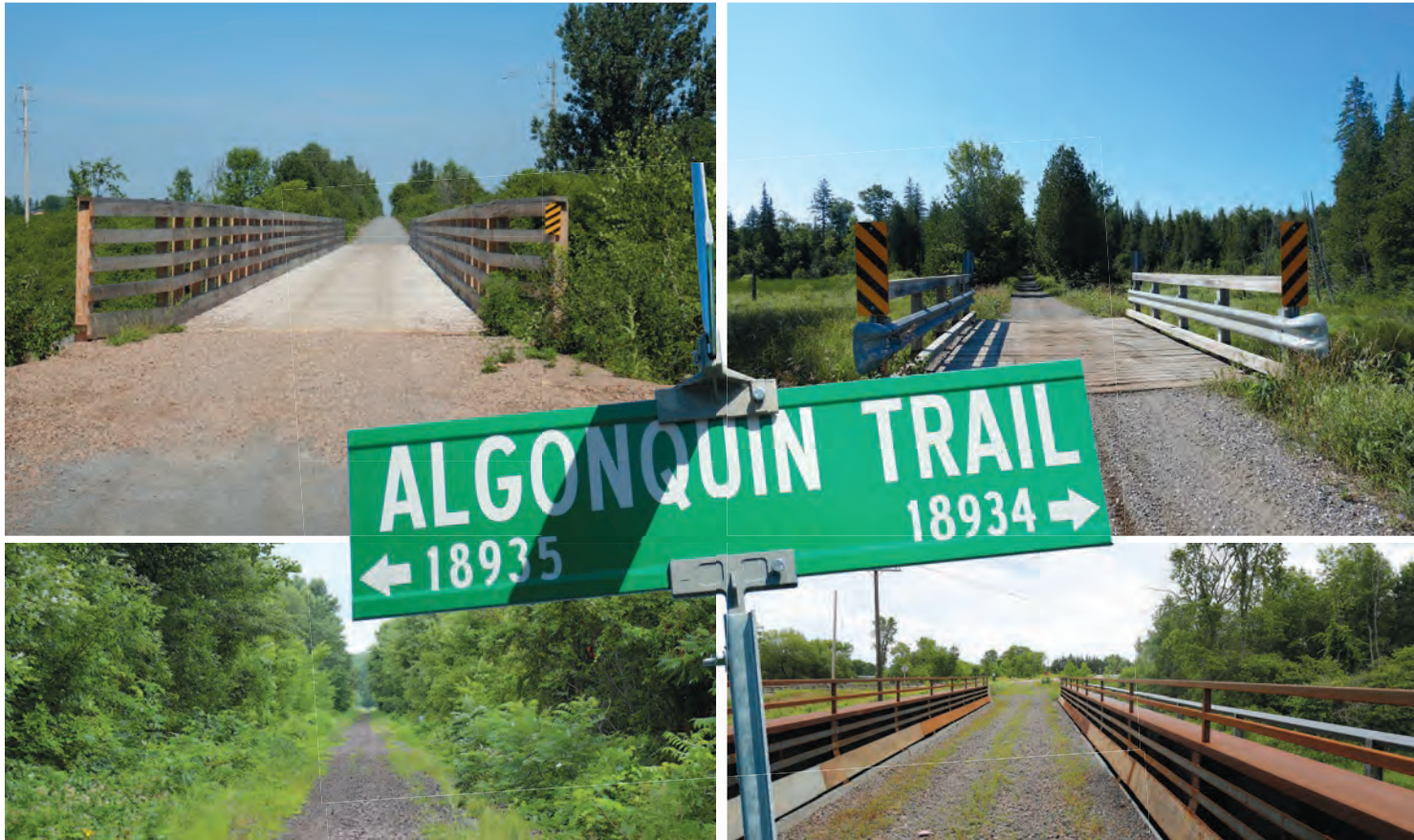
There is a lot of work to do on the trails, including 37 bridges and many underpasses that need to be made safe for everyone from cyclists to snowmobilers.
