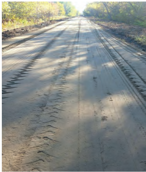
A section of the Ottawa Valley Rail Trail before and after road work was done. Although rail beds have a good base, once the rails are torn out the surface becomes very uneven and rail debris, including glass needs to be cleaned up.
