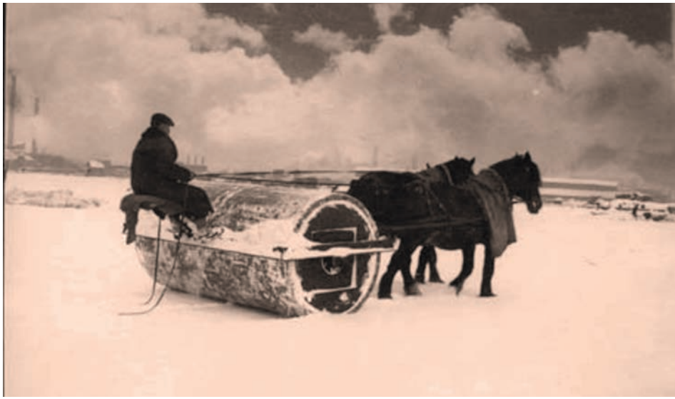
Horse drawn snow rollers were used to pack down snow on the roads. Packed snow was needed for horse drawn sleighs and logging wagons. Snow wardens had to pack snow onto roads that passed inside covered bridges to keep the ride smooth. Ontario Archives photo by John Boyd, 1924, shows a roller on the Ottawa River to create a road for horse teams to haul logs on the ice.
