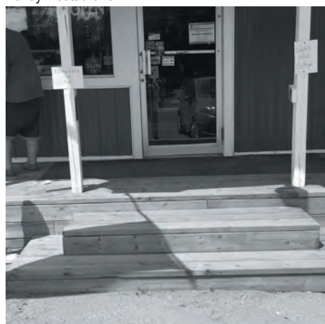
Nice job on the renovated entrance at the PVR!
