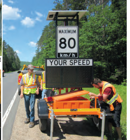
Installing the speed monitor on Hwy 41 in Griffith
