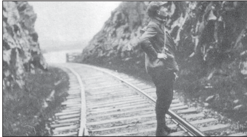
K & P rock cut at Bluff Point (Calabogie) 1912
