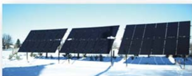
On the left: A partial shot of a 10kW Ground-Mounted system.
