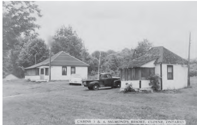
Cabins 3 and 4, Salmond's Resort. Main building, Bunkhouse, and long row of rooms for extra accommodation. Unknown date.
