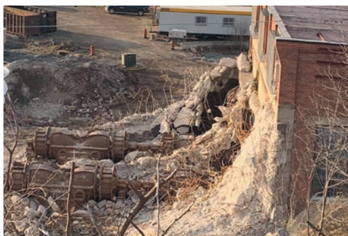
Work to dismantle and expand the OPG Generating station in Calabogie continued over the winter. Turbines that have been operating since 1914 were removed and shipped out. Pics by Nick Tourangeau and Jeff Levesque
