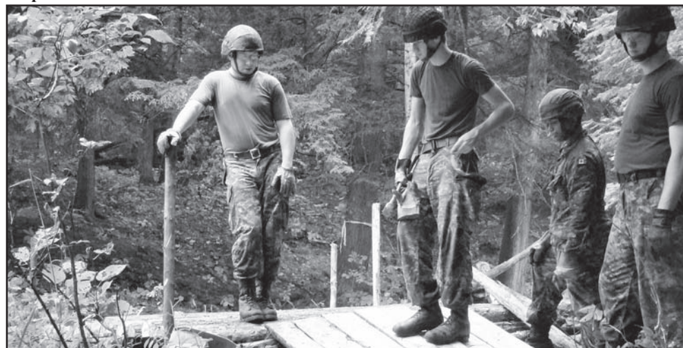
4 Troop reservists building a bridge
