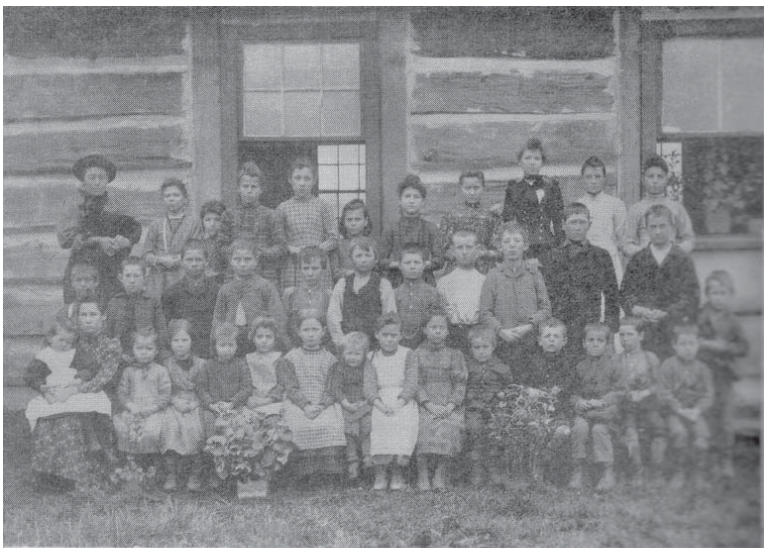
LOG SCHOOL HOUSE IN CAMEL CHUTE (1896)
