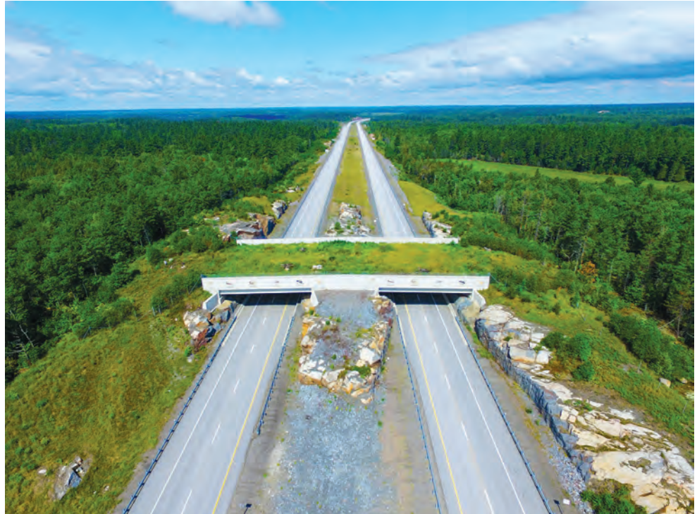
The Ontario overpass for wildlife was completed in 2012. It's south of Sudbury and was installed in this location due to the high number of moose and vehicle collisions. Credit: Ontario Ministry of Transportation
