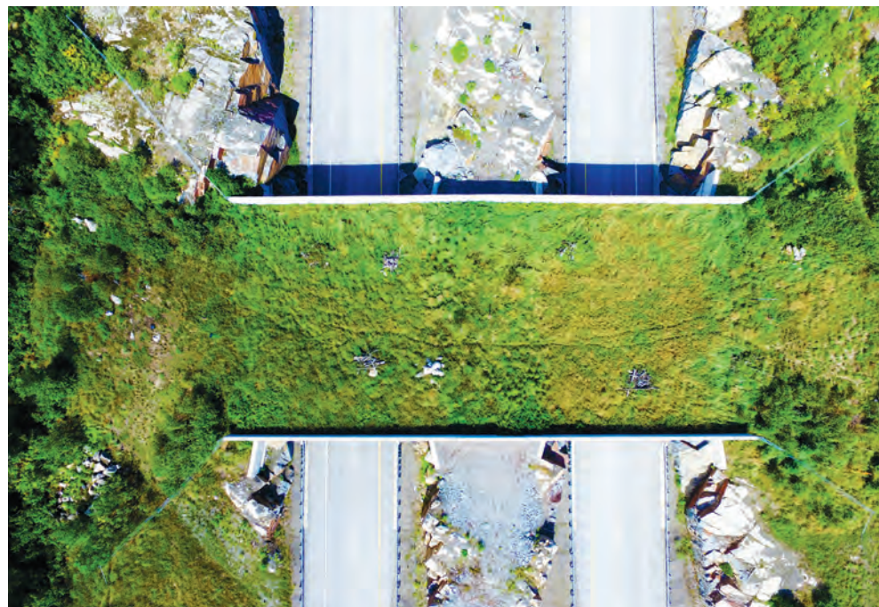
Even before the overpass was fully completed and six kilometres of fencing installed to help direct wildlife to the overpass, several animals were using it to cross over the highway. Credit: Ontario Ministry of Transportation
