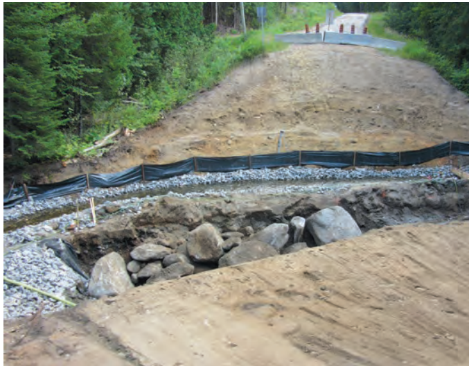
The Matawatchan Road is closed while the large culvert is being replaced by a bridge over Colton Creek. The workers had to divert the stream before digging to remove the culvert. If all goes well the bridge should be completed and the road will be open by the end of September. Traffic has been diverted down the narrow Frontenac Road in the meantime.
