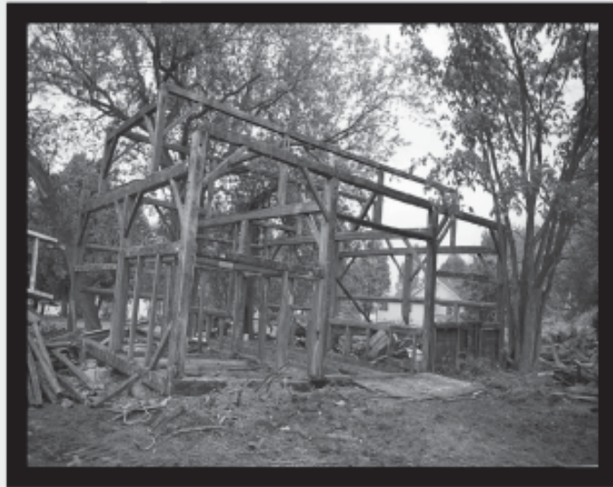
An 1800's barn restoration project underway
