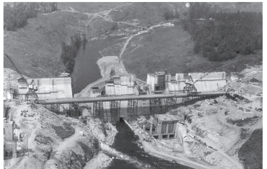
Mountain Chute Generating Station, 1965
