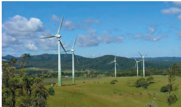
Wind farm in Queensland Australia. Straight lines of towers reduce infrastructure costs. (image thebackshed.com)
