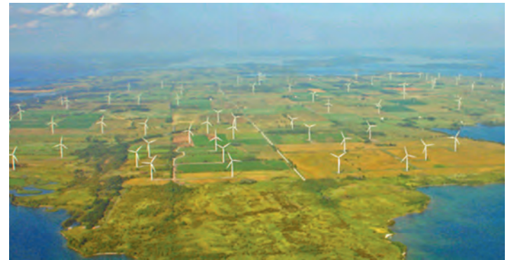
Wolfe Island from the air. Dense clustering reduces developers' infrastructure costs, with distance needed for unobstructed air flow. (image soundmann.com)
