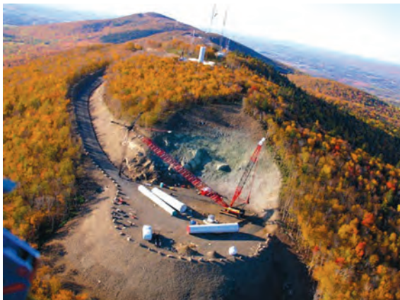
Construction Mars Hill, Maine. A level surface is needed. Roads must be capable of moving heavy vehicles carrying loads up to 50 meters long. vermonterswithvision.org
