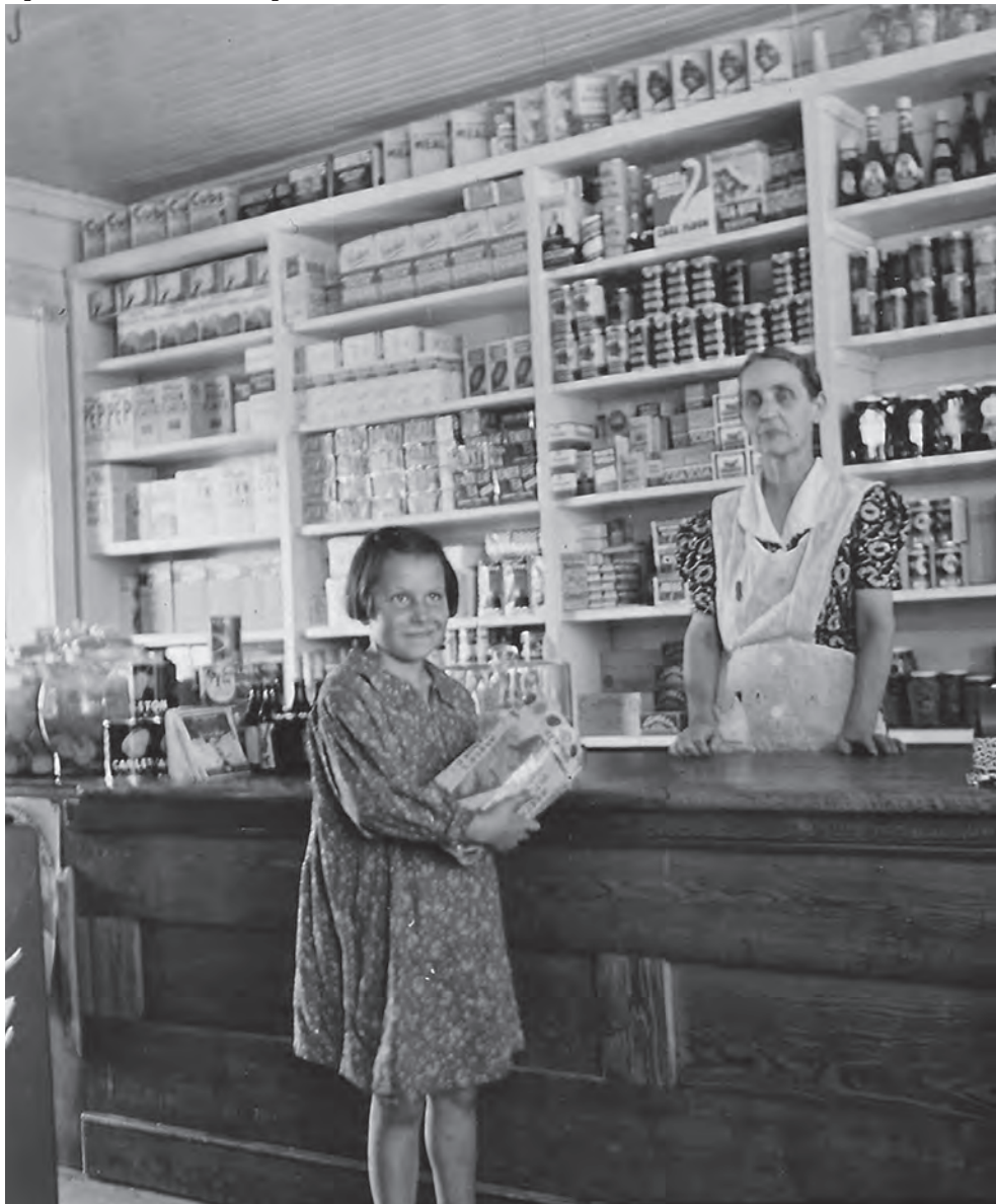
Glaeser's General Store is located in Denbigh. The store was first established in the early 1900s by Herman Glaeser and was owned and operated by descendants of the family as a central Denbigh location to stock up on 'everything'. The store was purchased and reopened in May 2014 by Peter and Karen Lips and is called 'Glaeser's Country Store'. Information sourced from: www.glaeserscs.com The young girl in the photo is Grace Glaeser (Kenny). She is the niece of the owner of the store, Adolf Glaeser. Photo taken around 1936. Part of the Peter and Mary Jane Turner Collection
