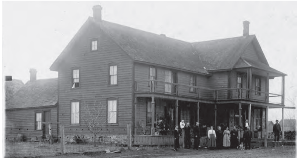
Flinton Store - September 1913 From the Alkenbrack album. The back inscription reads: 'Where Claude was born 1889. My father and uncle built this house while in partnership. This house is all grouted with mortar and the shingles were laid in mortar. The baby of the post is Douglas Alkenbrack taken September 1913. His father is holding him.'
