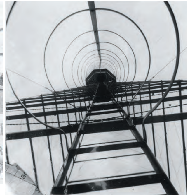
Looking Up The Ladder - Myer's Cave Fire Tower
