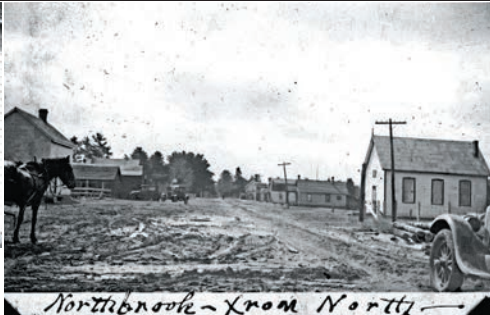
Right: Methodist Church, which is still standing. It has served as a drop-off location for used clothing for the community and is operated by the United Church of Canada. In the background, on the right, is Thompson's Store.
