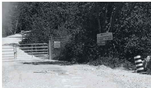
The road to the OPG is closed and adorned with No Trespassing signs as construction begins on a new generating station in Calabogie.
