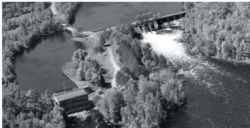
The 103 year old Ontario Power Corporation Generating Station in Calabogie produces half of the power the new generating station will produce starting some time in 2022.
